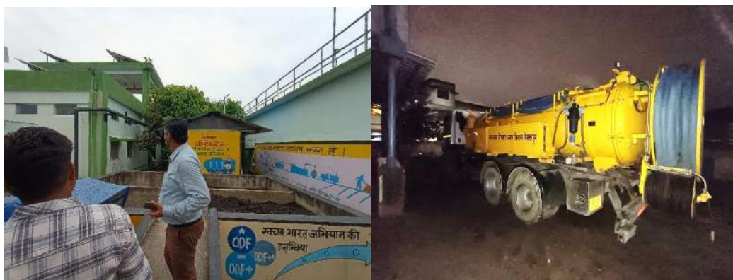
Image 4-1: 50 KLD Co-treatment plant at Gorakhpur Zoo and Mobile FSM Vehicle at Mahewa Mandi
