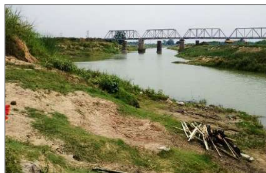
Image 6-17: Degraded Riparian stretches at Rohini River near Sitkaur
