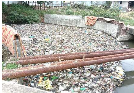
Image 6-2: Solid waste accumulation at Paidleganj Nallah at Buddha Gate
