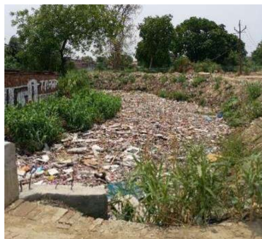
Image 4-4: Solid waste accumulated in Domingarh Drain near Rohini river.
