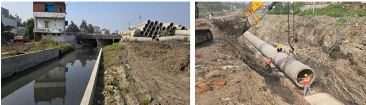
Image 6-13: Channelization of the Gurdahiya nallah and laying of sewer lines
