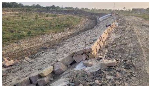
Image 6-23: Roadworks and stone pitching works at the Ekla Bandha site
