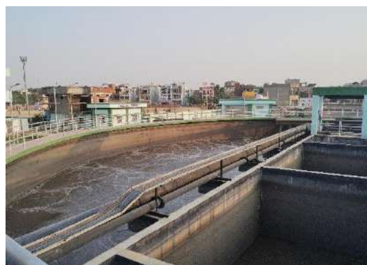
10 MLD STP at Subash Chandra Bose Nagar
