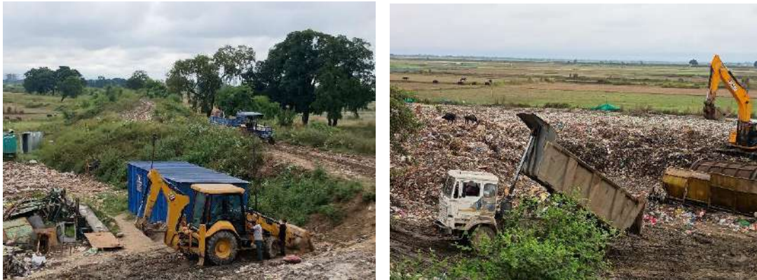
Image 4-2: Temporary Dump Site at Zero Point, Sahjanwa, Gorakhpur
