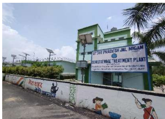
30 MLD STP at Gorakhpur Zoo
